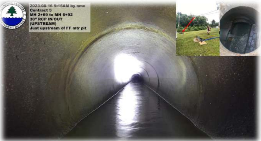
Pipe Inspection With New Pole Camera
